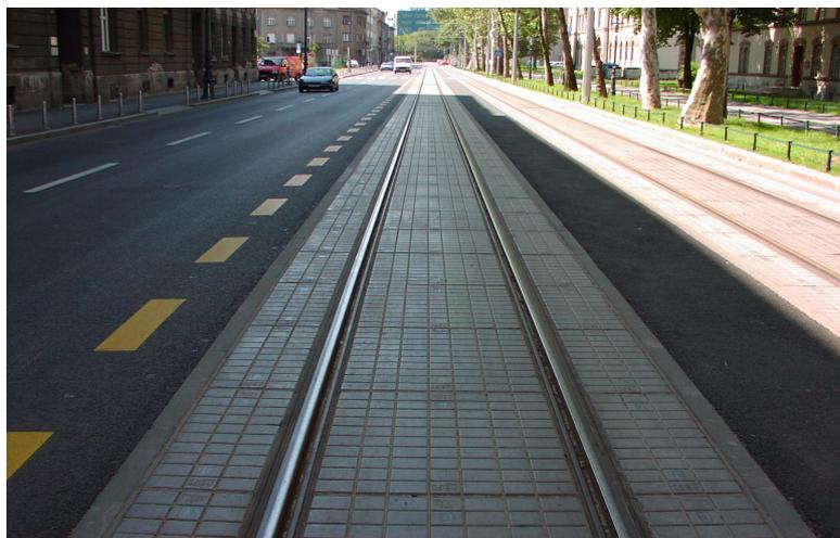
DEPP track fastening system has been in use since 1997 as a standard solution for the light rail and tram tracks in Croatia. Until today there have been installed over 80.000 DEPP type fastening points on tram tracks in Zagreb and Osijek, without any problems or objections.
